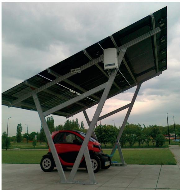
Fig. 2. Photovoltaic carport used to charge electric vehicles
