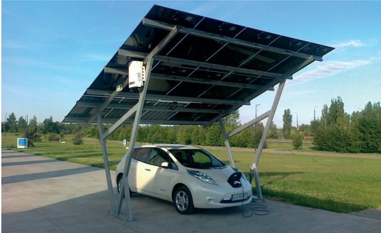
Fig. 7. An electric car during charging from carport
